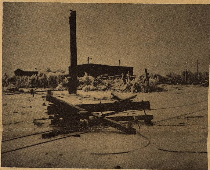
DOWNED POWER LINE ON PLAINS
