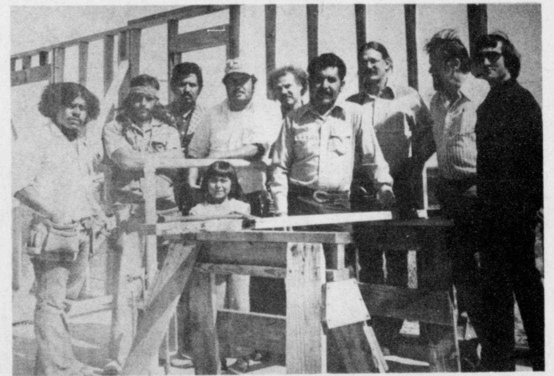
HOUSING VIPs IN TOWN . . . Clay C. Cochran and David Raphael, national housing experts were in Muleshoe for a two-day consultation and review session, Friday, September 26. They are shown looking over one of the housing units being constructed at this time. (l-r) Ray Costilla, Thomas Gonzales, Raymond Cabrera, Manuel Pineda, Rachel Pineda, David Raphael, Washington; David Quick, Clay Cochran, Washington; and Marcus Puente. Those persons shown with the two men from Washington are staff members or participants of the self-help housing project in Muleshoe.
