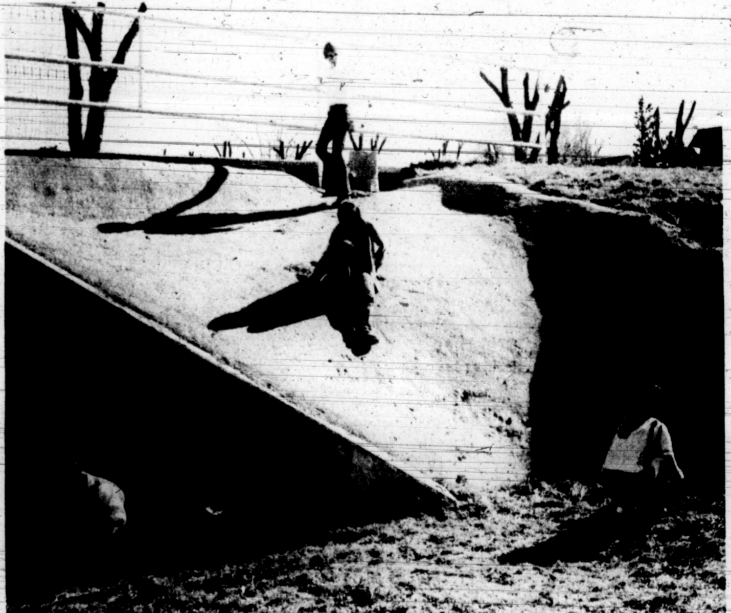
ON THE RAMP from the bridge, club members clean up material that has accumulated on the concrete. Members are Brian Thornton, top, and
