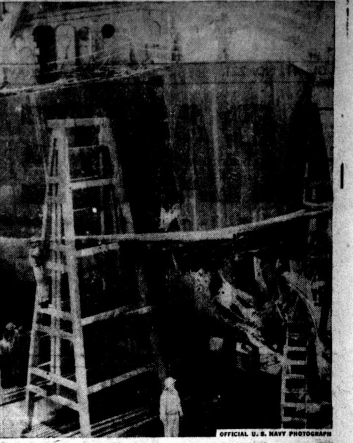
The bow of this old four-stake destroyer was blasted off in the Caribbean by a U-boat's torpedo. Prompt repairs at sea by a Ship Repair Unit kept her from sinking, enabling her to limp under her own power to a Navy Yard for permanent repairs. There she was fitted with a new bow from a decommissioned ship and sent back into action. It's for emergency jobs like this that the Navy needs men for the SRU's. Petty Officer ratings, with base pay from $78 to $126, plus 20 per cent for overseas service, may be given to qualified skilled craftsmen. Complete information is available at the Navy Recruiting Station.
