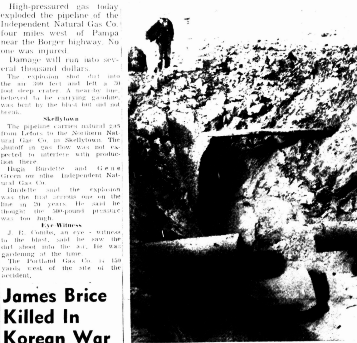
GAS EXPLODES — High-pressure gas ripped a hole in the pipeline of the Independent Natural Gas Co. west of Pampa this morning. Escaping gas and repairs to the line will cost several thousand dollars. No one was injured. Line in background was bent but was not broken. (News Photo)
