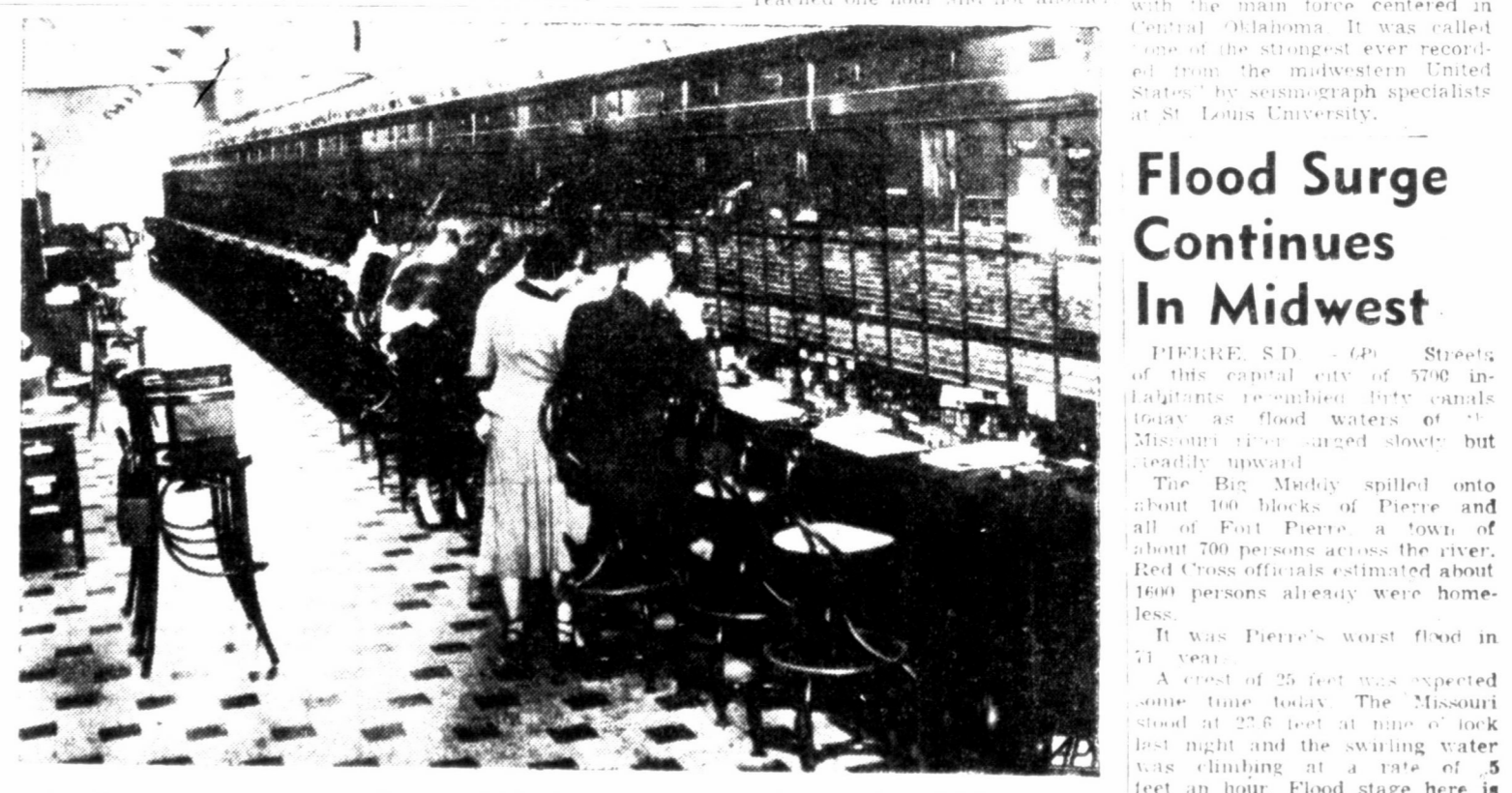
MAN SWITCHBOARDS — A small group of telephone company supervisors try to maintain service at one of the long distance switchboards where 40 operators usually are at work. No walkoff has been reported here in Pampa. (AP Wirephoto)
