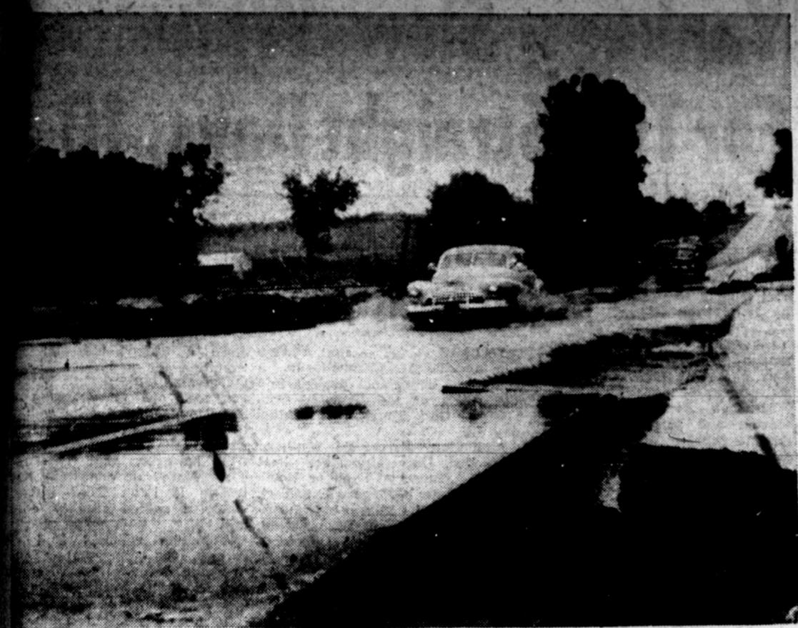
RAIN VICTIM — The road above, Highway 83 between Wheeler and Canadian, is one of the primary headaches confronting highway workmen. The road was badly undermined after heavy rains burst a stock tank dam near Wheeler and emptied the tank over the highway. The break is about two miles north of Wheeler. (News Engraving)
