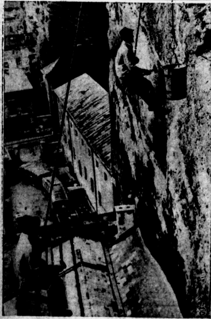
"MOUNTAIN CLEANERS" AT WORK—Working in much the same manner as our city window-cleaners—except with hammers—these "mountain cleaners" at Salzburg, Austria, work on the sides of sheer cliffs above the town. Their job each spring is to check the walls for loosened stones that may endanger life and property below.
