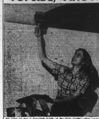
It's wise to use a four-inch brush of the best quality when you're painting a ceiling. If your brush is dry before you dip it into the paint the first time, it will help to minimize spattering. Keep the handle of your brush wiped dry for the same reason. Work across the narrow dimension of the room and paint a strip no more than two feet wide, at one time—so the edge won't dry before you start the next lap. The ceiling should, of course, be done before the walls.
