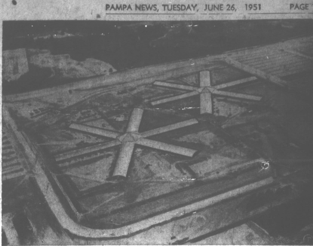
H-BOMB STARS ON THE SAVANNAH—An aerial view of the Savannah River atomic energy plant near Ellerton, S. C., shows the star-shaped construction of administration buildings of the Atomic Energy Commission and the DuPont Company. Built of steel and concrete, the building's wings measure 300 by 60 feet. The Savannah plant will be equipped much like the atomic energy plant at Hanford, Wash., with the additional capacity of working on hydrogen bombs.
