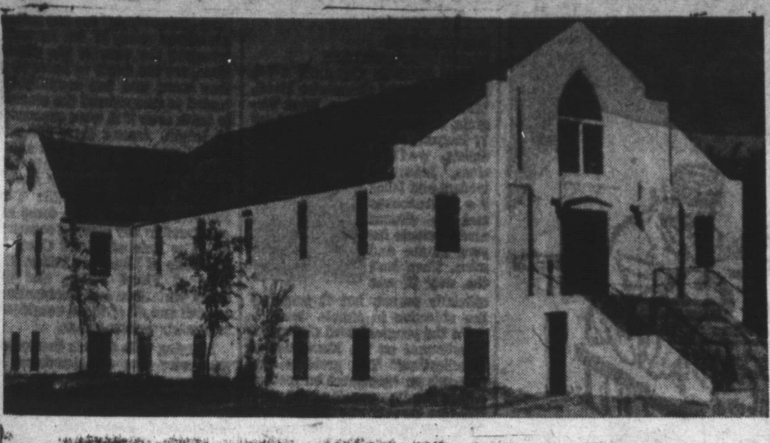
DEDICATION — The Methodist Church of Lefors, completed in 1948, will be dedicated Sunday. The church was constructed during the pastorate of the Rev. N. S. Daniel. It is valued at $30,000, which includes furnishings. The Rev. W. E. Hamilton, Methodist district superintendent, will officiate. The Rev. Walter V. O'Kelly is pastor of the church.
