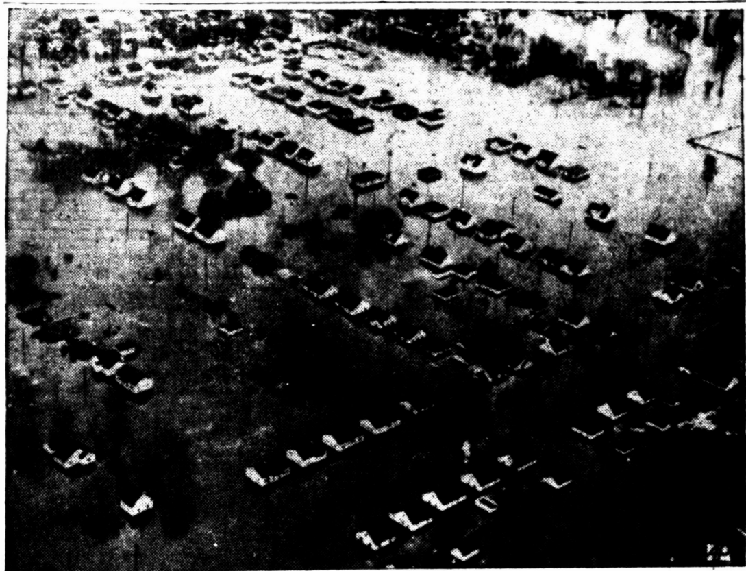
FLOOD ENIGNS HOUSES — Flood waters from the usually placid and relatively small Minnesota river at Mankato, Minn., laps above the first floors of hundreds of homes in a suburban area April 9. Residents in the area were evacuated as waters from tributary streams continued to pour into the river. (AP Wirephoto)
