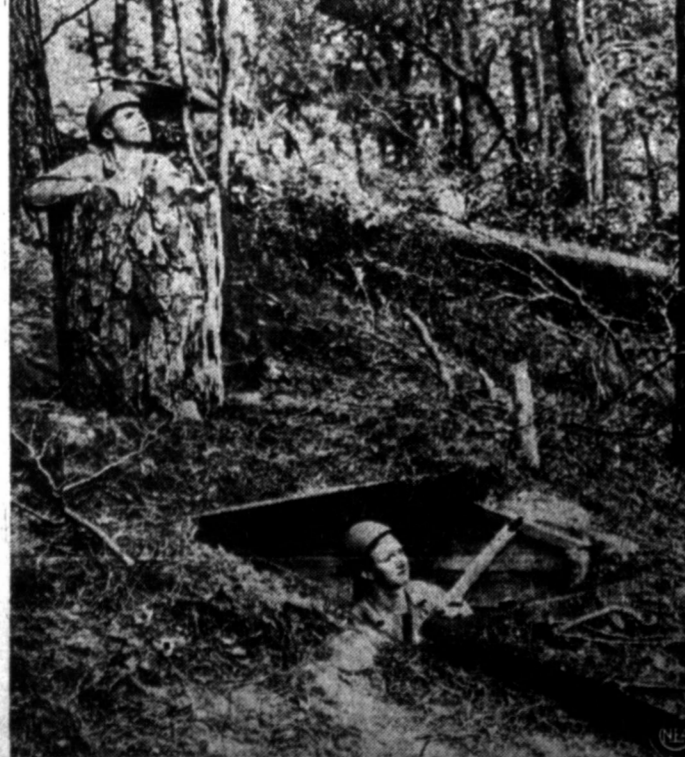
It looks like the funny papers, but it's grim business for these Navy Construction Battalion members training for war at Camp Peary, Va. Like these two Seabees in a camouflaged machine gun nest, all Seabees must know how to fight as well as work when sent overseas to build outlying bases.
