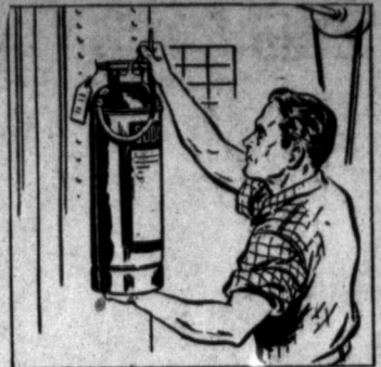
Grasp nozzle of soda acid or foam extinguisher before lifting from the wall bracket.
