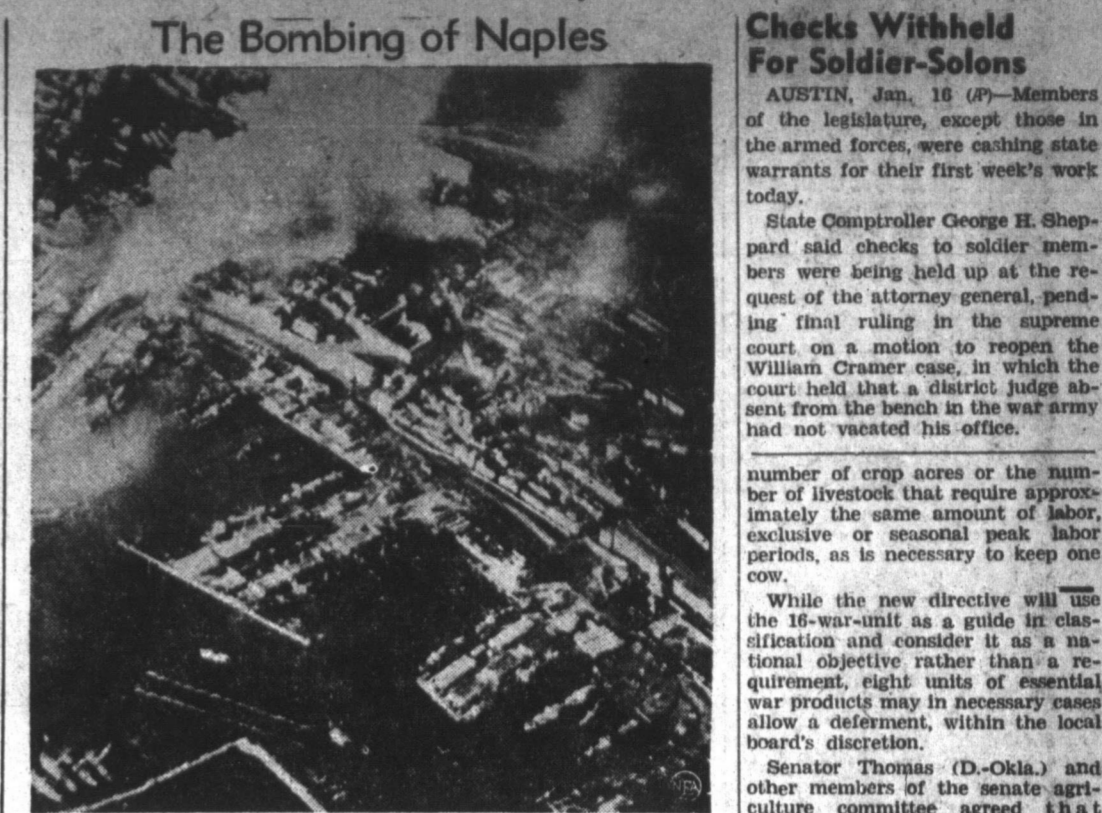
Airview from an American Army plane shows fires burning in the dock sections of Naples, Italy, after a U. S. raid on that important supply port for the axis armies in Tunisia.
