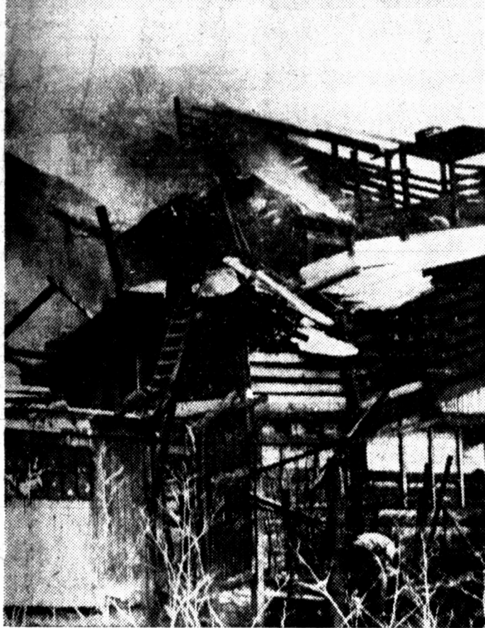
Shown is the fire gutted building of the Frye Meat Packers of Seattle, Wash., where 28 persons were killed. The Boeing bomber, one engine afire during a test flight, smashed into the plant spreading flaming death and destruction throughout the building. The wreckage of the plane is in the above building. (NEA TELEPHOTO)
