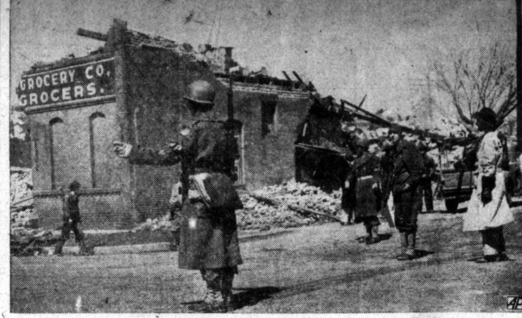
A mile-wide tornado, which killed one person and injured five, damaged about 80 per cent of the business houses and homes and almost demolished this grocery company warehouse at San Augustine, Tex. Soldiers are shown helping police streets as residents bend to the work of salvage.
