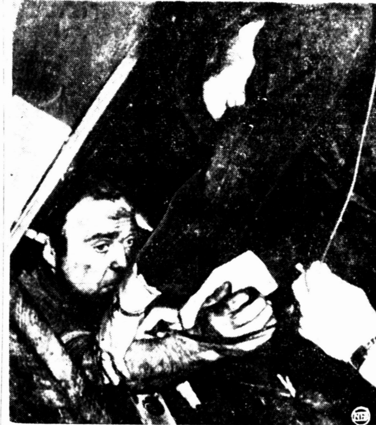
Trapped when two floors of a warehouse collapsed in Little Falls, N. Y., Carl Vogt, 37, is given a blood transfusion by Dr. Ray Knowles as the victim still lies pinned in wreckage. Three were crushed to death and two others hurt.
