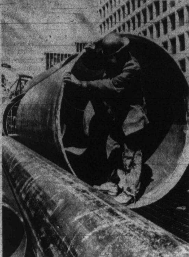
THE UNDERGROUND is exposed in Washington as this workman makes a final inspection on Fiberglas-reinforced plastic sewer pipe. These 20-foot sections replace some pipe in use since the British burned the capital in 1814.
