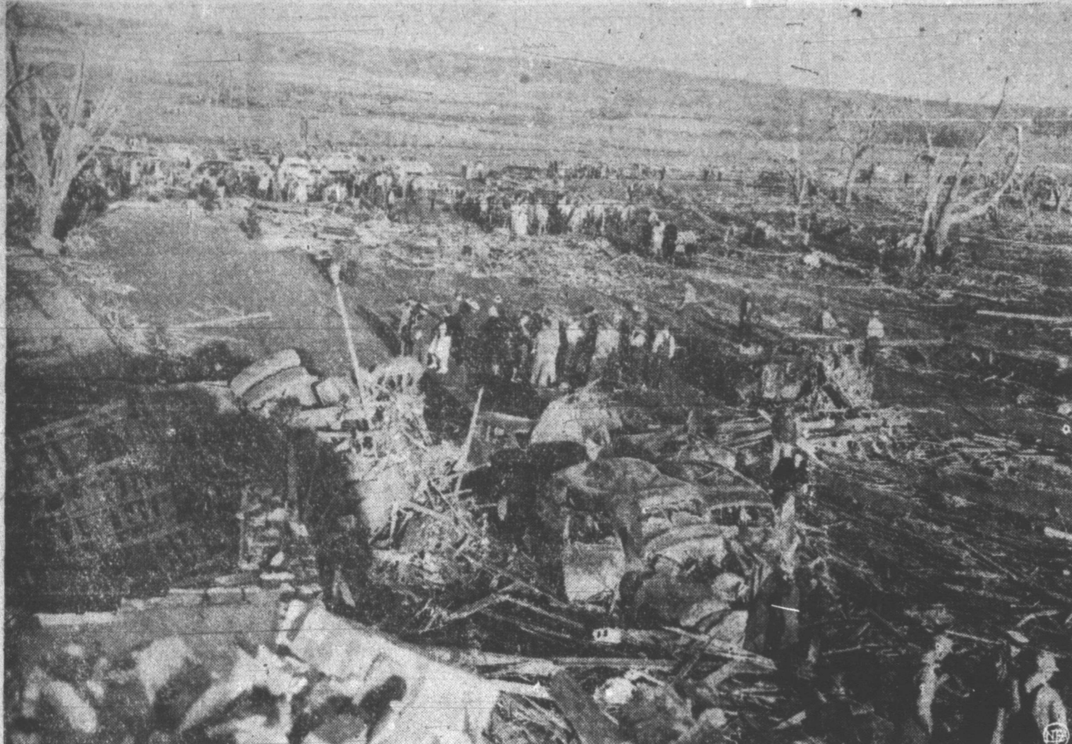
TORNADO CRUSHES MISSOURI TOWN —This is a general view of downtown Worth, Mo., after the village of 233 persons was struck by a tornado. Twenty persons were killed, eight were dangerously injured and forty persons received minor injuries in the storm.
