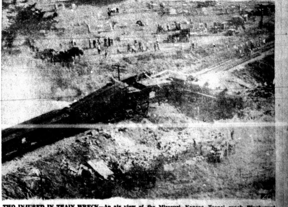
TWO INJURED IN TRAIN WRECK—An air view of the Missouri-Kansas-Texas' crack Bluebonnet Special, running from Kansas City to Dallas, which derailed near Leonard, Texas, after plunging into the rear of a slow-moving freight during a dense, early morning fog. Two train crewmen were injured. The wreck occurred in the Leonard Cemetery through which the railroad passes.
