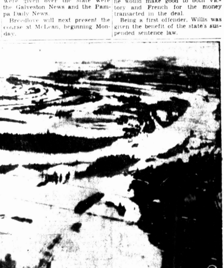
RAINS FLOOD OREGON STREAMS—This aerial view shows the flooded Willamette River Valley at Independence, Ore., right. The pattern in the foreground is caused by wire support poles in the hop yards which are numerous in this area. The flood, caused by heavy rains, disrupted transportation and forced hundreds of families from their homes.
