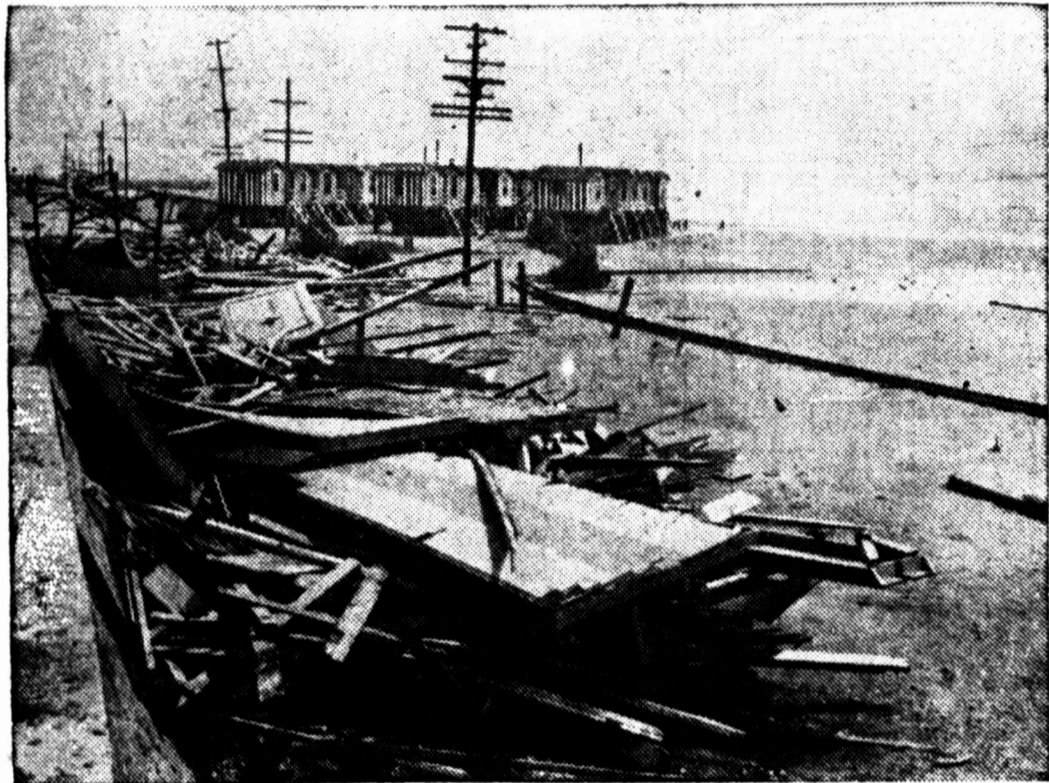
GALVESTON STORM DAMAGE —This is the East Beach at Galveston where the city operated playground consisting of swings, a miniature railroad named Tootsie after Phil Harris and Alice Faye's baby, and other rides, lies smashed to bits against the sea wall. The bath houses in the background withstood the storm with minor damage.
