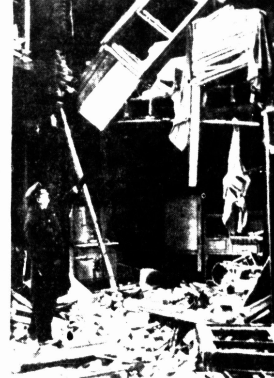
EXPLOSION WRECKS HOME—Three persons were injured in a gas explosion which left their Pittsburgh, Pa., home, shown here, badly damaged. One of the injured was pinned under debris for a half hour before being rescued by firemen. Loss was estimated at $2,500.
