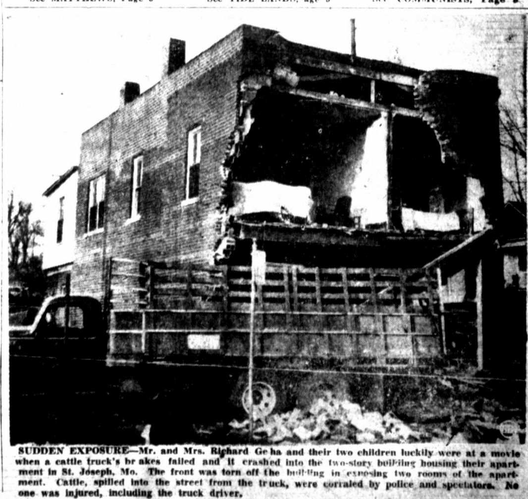
SUDDEN EXPOSURE—Mrs. and Mr. Richard Geha and their two children luckily were at a movie when a cattle truck's brakes failed and it crashed into the two-story building housing their apartment in St. Joseph, Mo. The front was torn off the building in exposing two rooms of the apartment. Cattle, spilled into the street from the truck, were corralled by police and spectators. No one was injured, including the truck driver.
