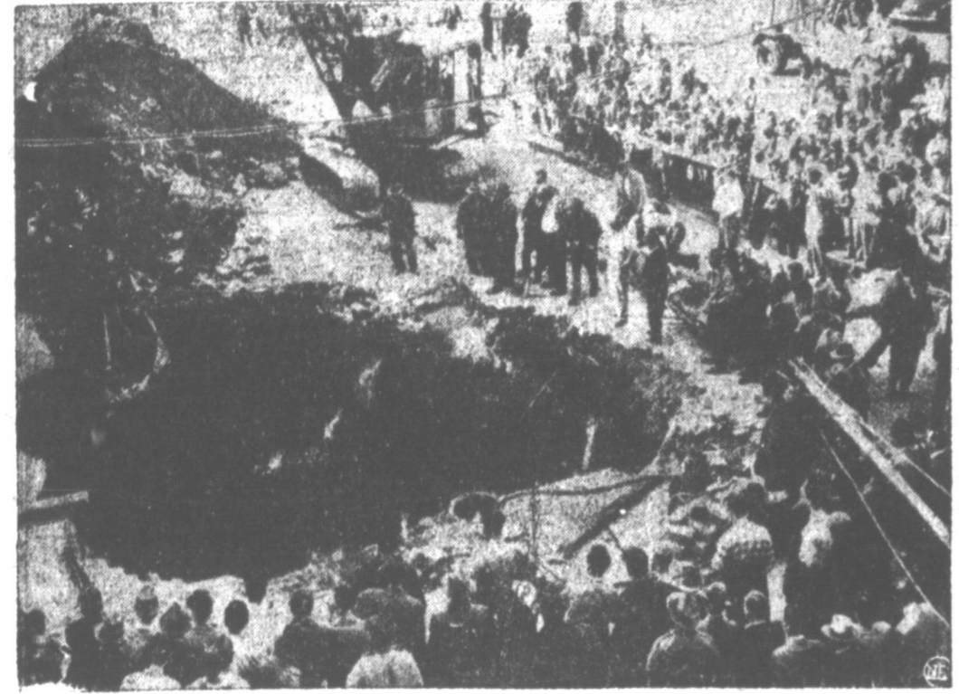
TRY TO FIND BODY IN CAVE-IN—Emergency crews work in a vain attempt to extricate the body of Angelo Corino, 35, water department employe, buried in a cave-in in Chelsea, Mass. Spectators watch as operation of a power shovel proved futile when sides of the hole, 30 feet square, kept caving in and filling the excavation.
