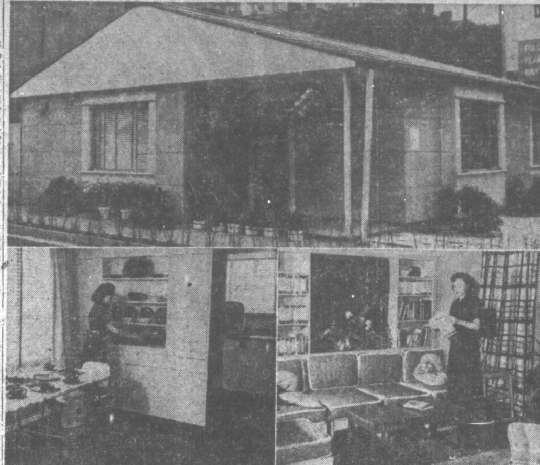
Five-room, all-steel porcelain enamel house, above, is fireproof and rustproof. Manufacturers claim the enamel finish which is used on both outdoor and indoor walls will never need repainting.
