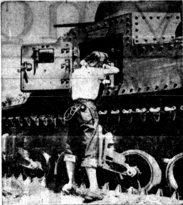
Feminine member of U. S. Army Signal Corps laboratories demonstrate correct method of installing radio set in tank.
