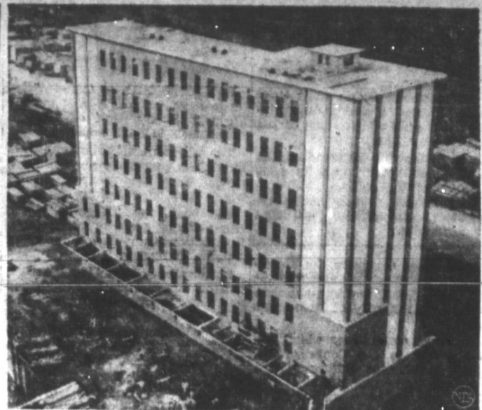
American funds are doing a big job in Europe, and here's a concrete example. This flour mill in Trieste was almost completely destroyed during the war, but U. S. aid funds rebuilt it into the largest and most modern plant of its kind in the Mediterranean area. It's now handling Marshall Plan flour for Trieste and Austria, and its silos hold 30,000 tons of grain.
