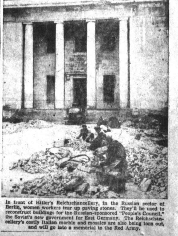
In front of Hitler's Reich Chancellery, in the Russian sector of Berlin, women workers tear up paving stones. They'll be used to reconstruct buildings for the Russian-sponsored 'People's Council,' the Soviet's new government for East Germany.
