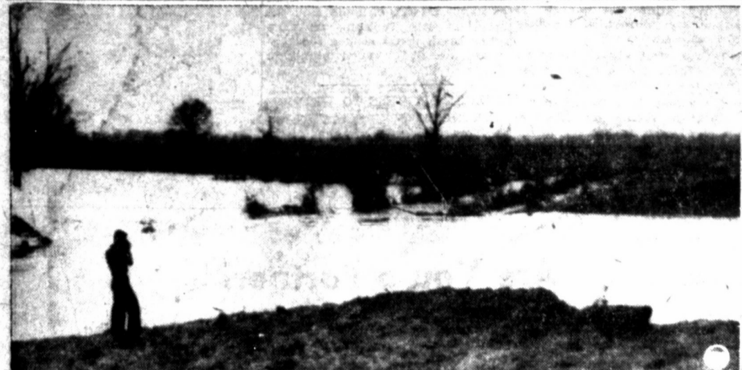
LEVEE BREAK—United States engineers are working to close this 229-foot crevasse at Port Allen, La., where water is pouring in from the Mississippi River levee. A spectator takes a picture of the break, which is about four miles north of Baton Rouge, capital of Louisiana, and across the river from that city. (NEA Telephoto)
