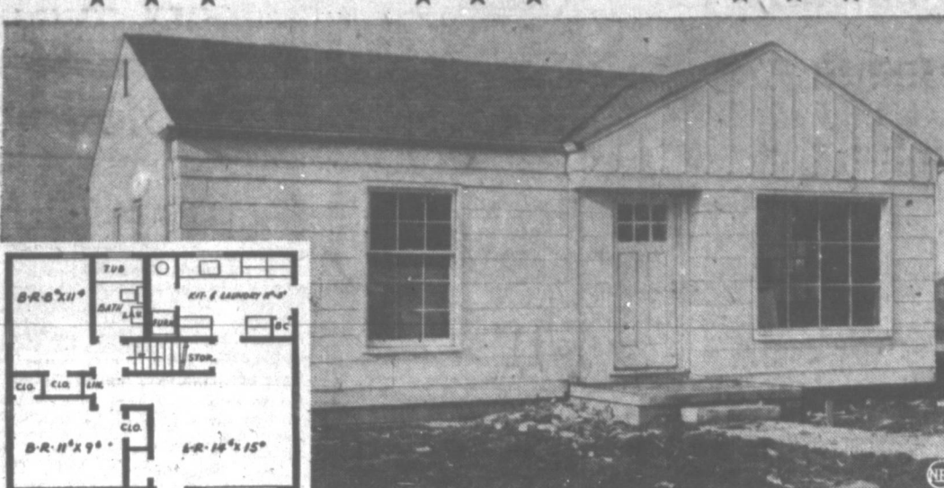
One of the 50 model low-cost homes in the demonstration being conducted by the Builders Association of Metropolitan Detroit, this two-bedroom house sells for $6,900, built on the buyer's own lot. Erected by R. M. Lockwood, president of the National Association of Home Builders, it could be expanded by adding a breezeway and connecting garage.
