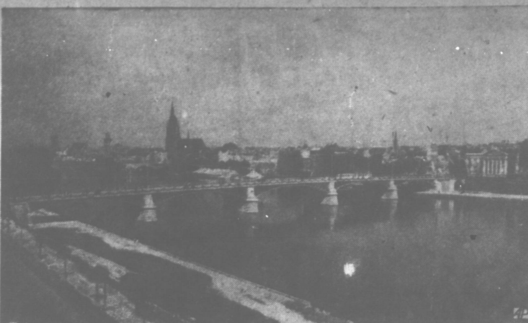
FRANKFURT REJOINED — Street car service between Central and South Frankfurt, Germany, was restored by the new Upper Main bridge. The cathedral is in the background.
