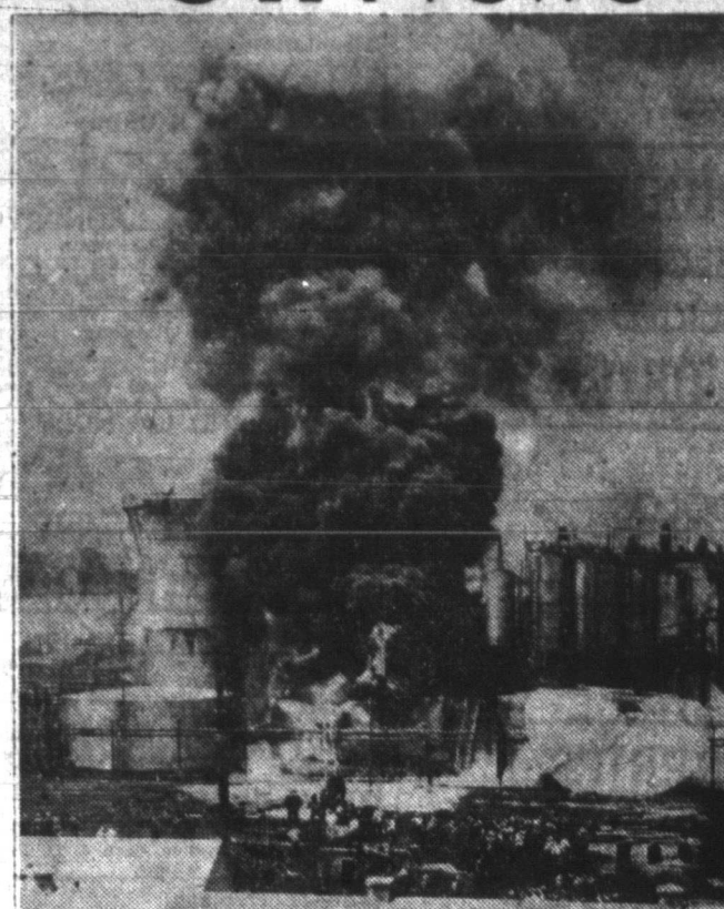
TANK FIRE THREATENS AREA—Dense smoke rises from a storage tank containing thousands of gallons of inflammable fluid after it ignited at the Gulf Refining Co. at Philadelphia. Flames soared more than 50 feet into the air as firemen fought to keep the fire from spreading to adjacent fuel oil tanks. The top of the tank is draped over another tank, at right, and firemen said it apparently was blown off the burning tank in the initial explosion. (AP Wirephoto)
