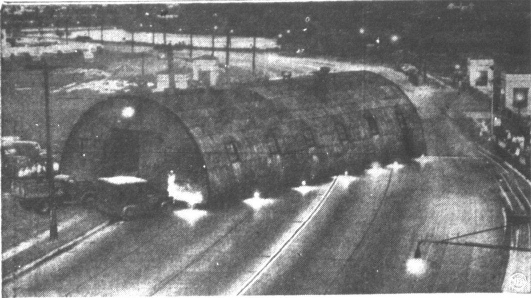
QUONSET HUT HITS THE ROAD—The owners of this 100-foot-long quonset hut, used as an auto body shop, needed it moved across the Cooper River at Camden, N. J. So they jacked it up on rollers and took it down the highway and ferried it across the stream. A dozen men completed the 300-yard road trip in less than an hour.
