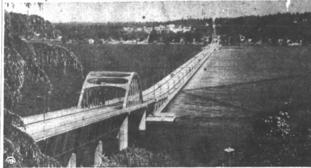
FLOATING BRIDGE—Connecting Seattle with the eastern shore of Puget Sound is the unique floating Lake Washington bridge. This view is looking from Seattle toward Mercer Island, the other terminus of the floating structure.
