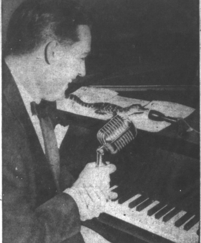
... AND GRASHING OF TEETH—Say your favorite quiz program is interrupted with a special bulletin: "And now we bring you as a public service the gnashing of a baby alligator's teeth." The chances are the station is testing a new type condenser microphone, a model of which is seen on the piano at right, alongside a conventional mike. The new mike has a range of 20 to 15,000 vibrations per second, far greater than types now in use. Orchestra leader Ray Harkett, above, at the Mark Hopkins Hotel in San Francisco, checks for himself the mike's ability to pick up an alligator's tooth-gnashing.
