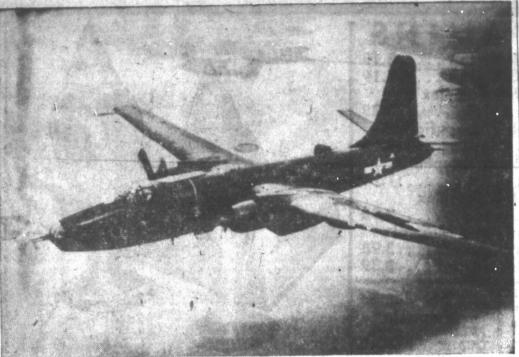
NAVY PLANE COMBINES JETS AND PROPS—This is the Navy's new patrol plane, the Martin P4M-1 Mercator, first shown to the public at the Cleveland Air Races. The aircraft has four engines but looks like a twin-engine model. Two standard gasoline engines are used for normal flight and the two jet engines, housed in the same nacelles, are used for extra bursts of speed. The Mercator is capable of speeds over 300 miles per hour and carries a load of 80,000 pounds.
