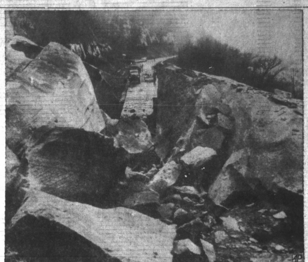
ROAD CLOSED—Tons of rock cover 200 feet of State Highway 7, Skyline Drive, near Marietta, Ohio. The rock slipped over the road, which was cut through almost solid rock a few years ago. No one was injured in the slide. Highway engineers said the road would be closed for two or three days. (AP Wirephoto)
