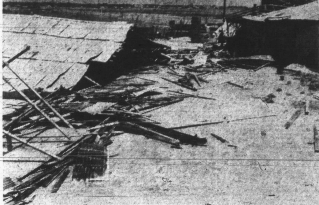
NEW SITE—Picked up by the heavy wind late Saturday night, this tanning barn owned by Arthur Reed was dropped on a new site some 40 to 50 feet south. Reed, whose home and business are located one-quarter mile outside the city limits on the Lefors Highway, says the estimated loss is $3,000. The concrete floor and foundation upon which the building rested can be seen in the background. (News Photo and Engraving)
