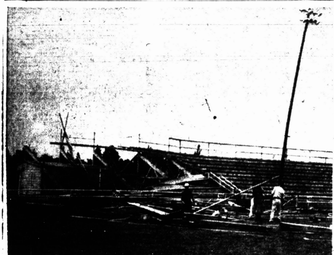
FOOTBALL FIELD HIT—A large part of this grandstand at Harvester football field was damaged by Saturday night's raging winds. School officials have not yet estimated the damage but it will probably run into the thousands of dollars. (News Photos and Engravings)
