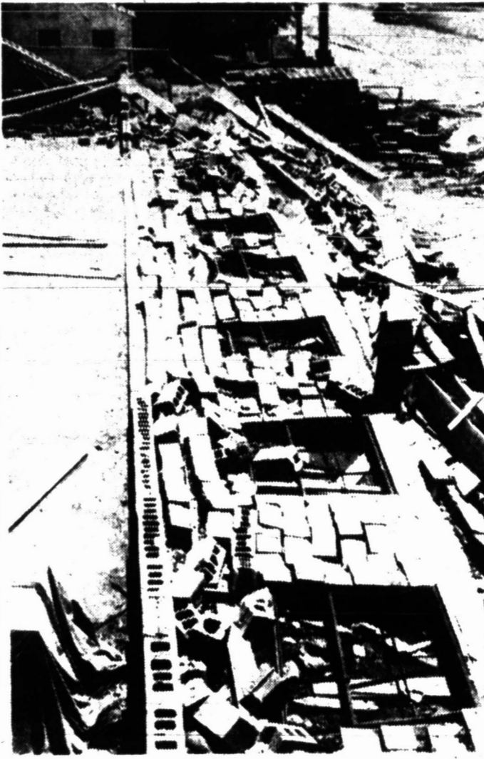
WALL COMES TUMBLING—What was a concrete wall being constructed at J. C. Daniels Motor Co. on West Tenth was a crumpled mass today after Saturday night's raging windstorm. Daniels estimated the loss at $3,000. (News Photos and Engravings)
