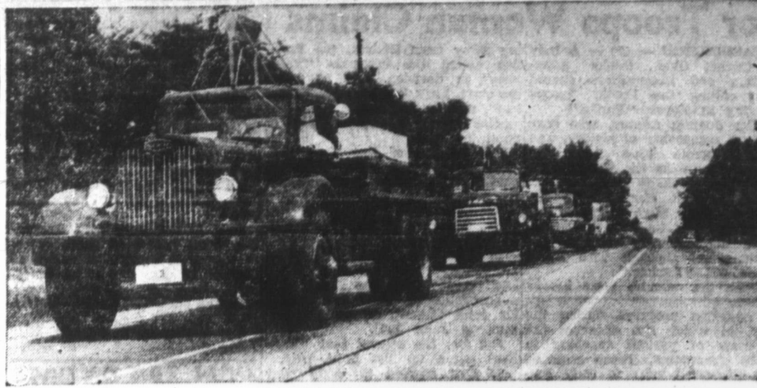
THREE-LANE TREADMILL — Day and night, these trucks will roll back and forth on a mile-long road in Maryland to see how much damage trucks do to highways.
