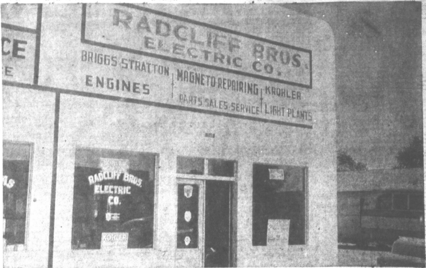
Radcliff Brothers Electric Company, a symbol of success in the electric field, have one of the outstanding electric supply houses in the Top o' Texas. From the smallest to the largest items in industrial and commercial needs, Radcliff has it. (News Photo and Engraving)
