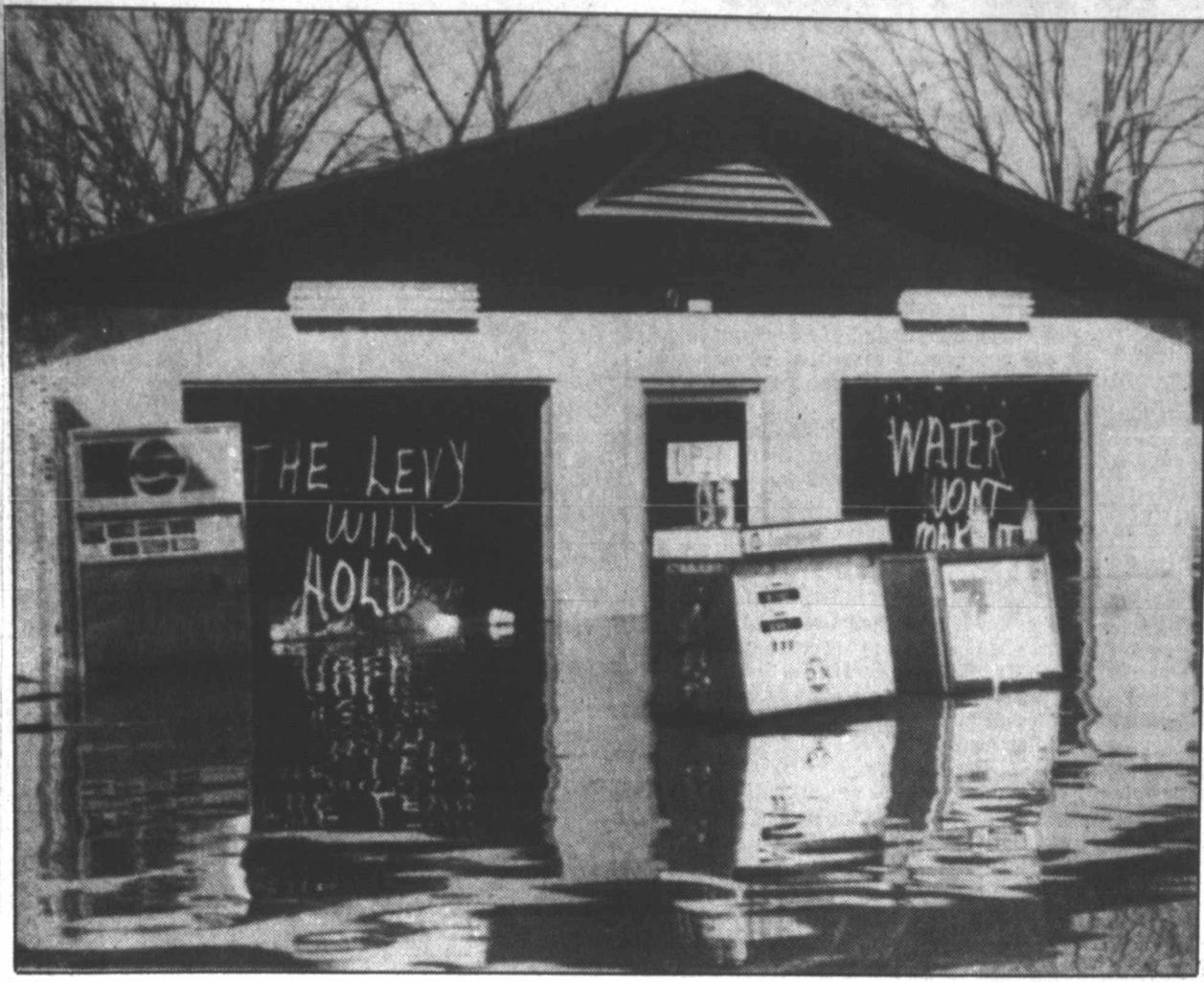
A Jacksonport, Ark. store and service station owner wrote "The levee will hold" on the window of his business, but the levee obviously did not hold, and the water made it. Flood waters covered the entire town. (AP Laserphoto)
