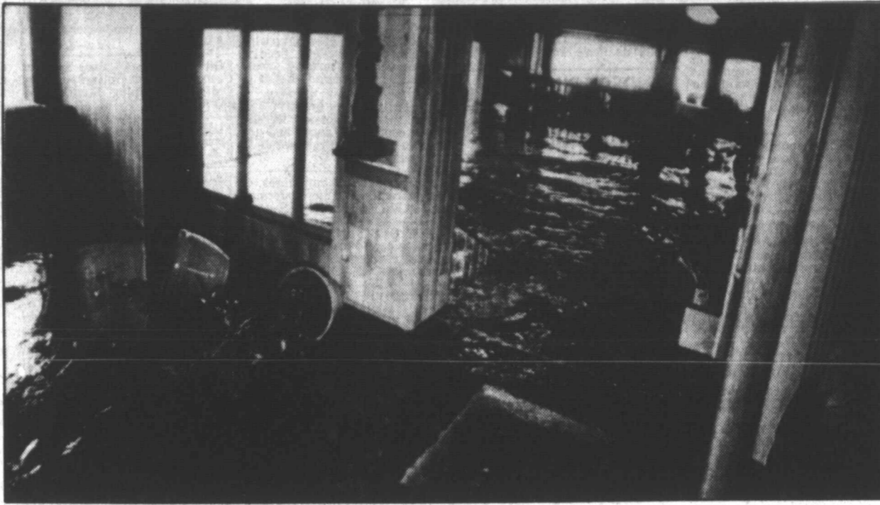
The Marine Room Restaurant of the La Jolla Beach and Tennis Club is washed out by heavy surf that broke through the walls Wednesday in La Jolla, Calif. The heavy surf was the result of a storm that pounded California Tuesday killing nine people. (AP Laserphoto)
