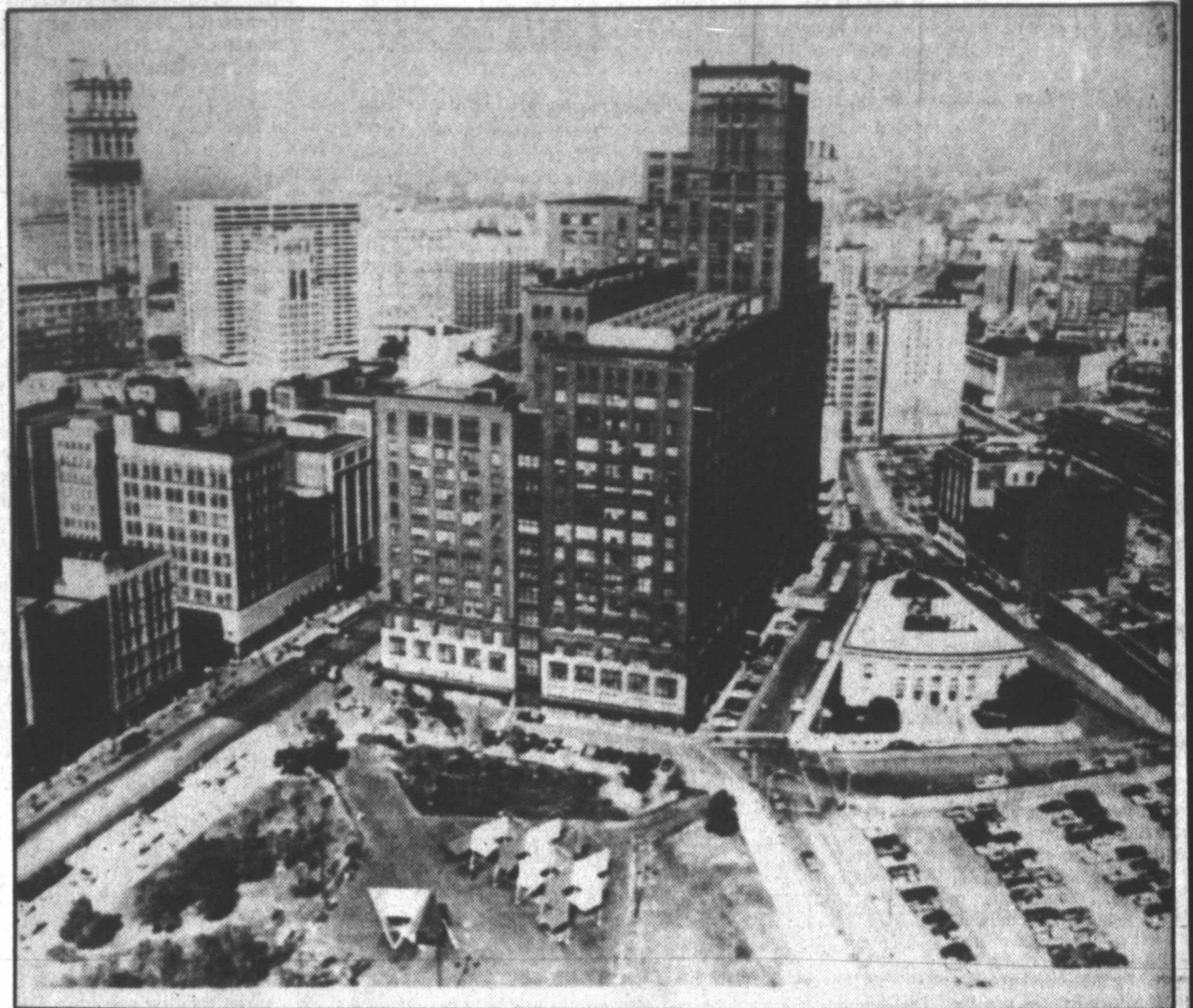
The J.L. Hudson's department store in downtown Detroit is scheduled to close at the end of the 1982 holiday shopping season. It is the last major retailer in the downtown area. This is an October 1982 picture. (AP Laserphoto)
