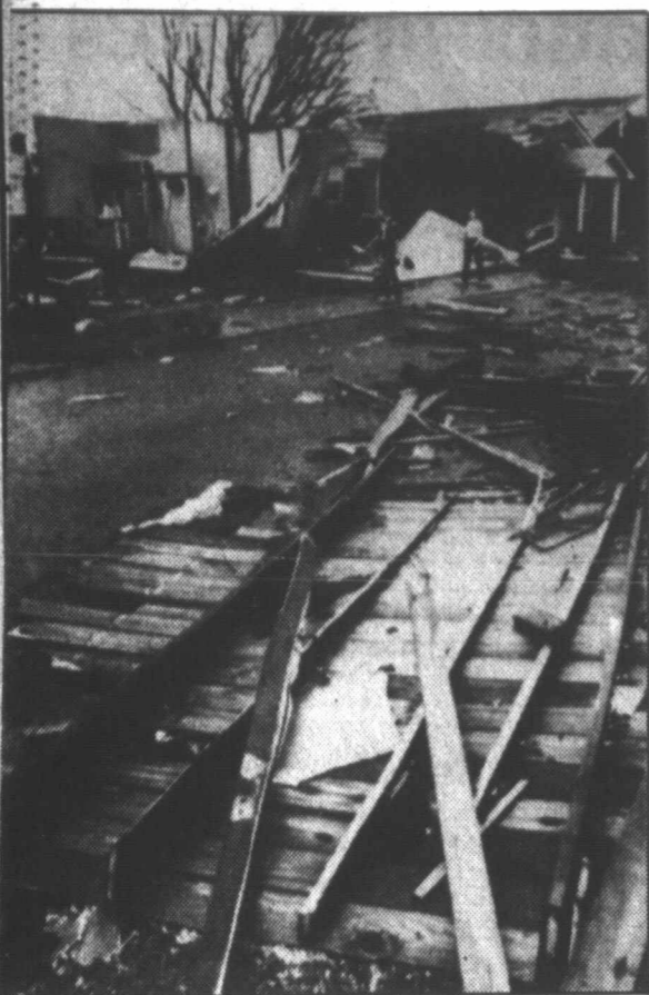
West Heights Baptist Church is in shambles Thursday after a storm struck the West Thirty-Fourth Street area of Little Rock, Ark. (AP Laserphoto)
