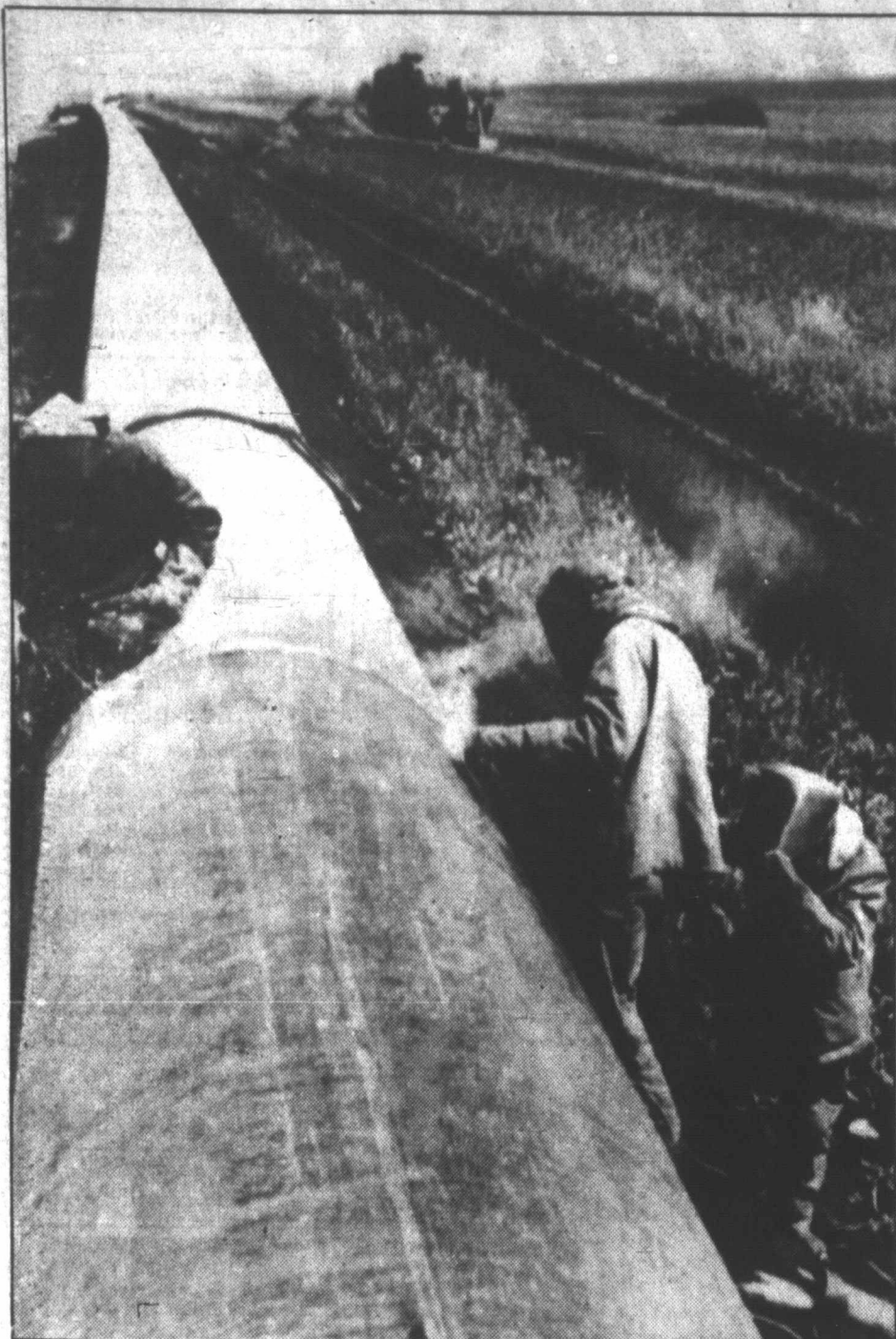
Soviet workers weld sections of the pipeline that will carry natural gas from the Soviet Union to western Europe. This section is in the Bashkir region. The United States has forbidden American technology from being exported by U.S. firms or their foreign subsidiaries for use in the pipeline. (AP Laserphoto)
