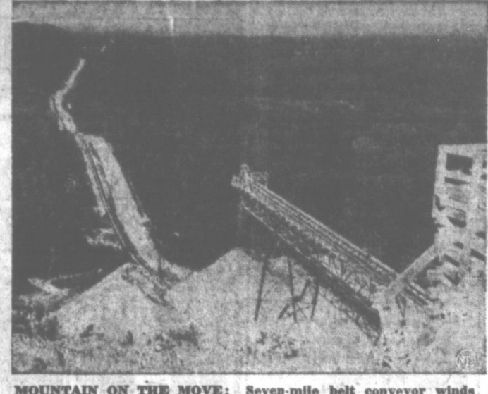
MOUNTAIN ON THE MOVE: Seven-mile belt conveyor winds through the Ozarks to carry four million tons of Lee Mountain across two valleys to the site of the Bull Shoals Dam.
