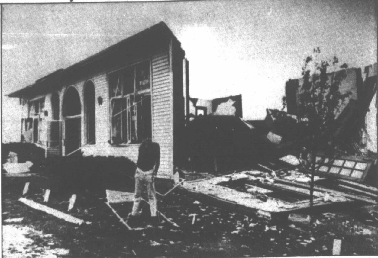
The 63-year-old Baptist Church in Mary, Illinois, was destroyed by heavy winds Tuesday which resulted in two deaths and millions of dollars in property damage in Central Illinois. Pastor Lon Simpson, standing in front of the rubble, watched the storm from the nearby parsonage. (AP Laserphoto)
