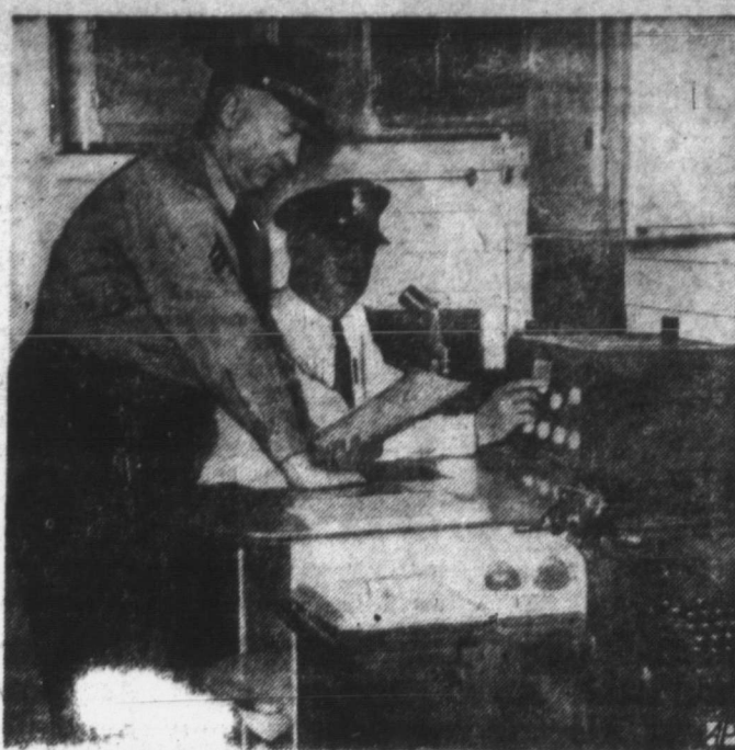
ROVING HEADQUARTERS — Sgt. William R. Lasham (left) and Inspector Mark Raspberry test radio in new mobile train headquarters for Washington, D. C. P. A. Police.
