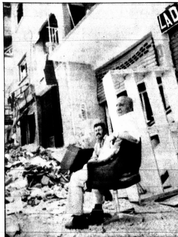
A Sidon shopowner sits outside the wreckage of his store in southern Lebanon Monday and contemplates what is left of his city. Reconstruction has not begun since the Israeli army stormed the city last month. (AP Laserphoto)
